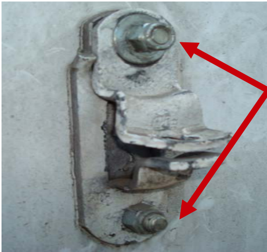
Different Bolts / Loosen Hasp
